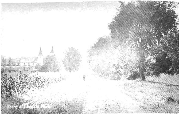
'Scene at Elmdale' - About 1910 - Highway 238 looking east.
